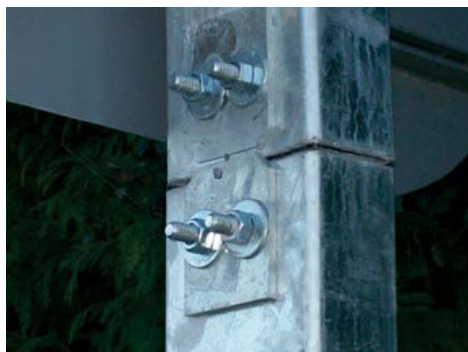
Figure 37: Breakaway/spliced pole ( left ) and slip base ( right ) [57]
