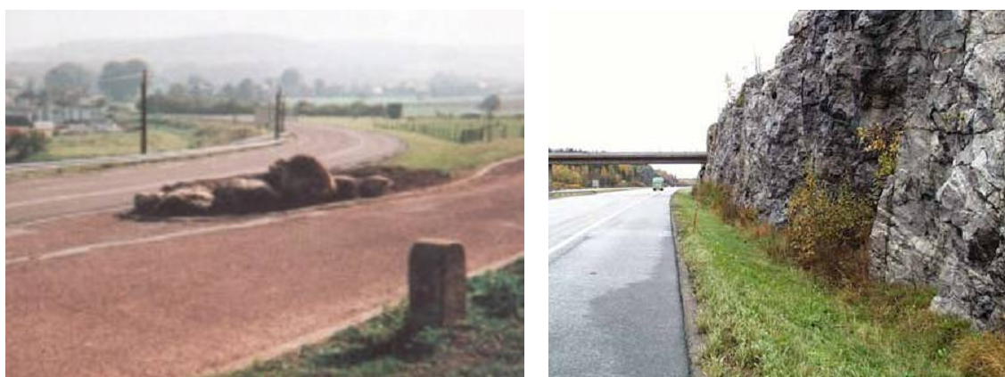
Figure 54: Examples of hazardous boulders ( left ) and rocks ( right ) on the roadside (Source: [A.2] and [A.3])
