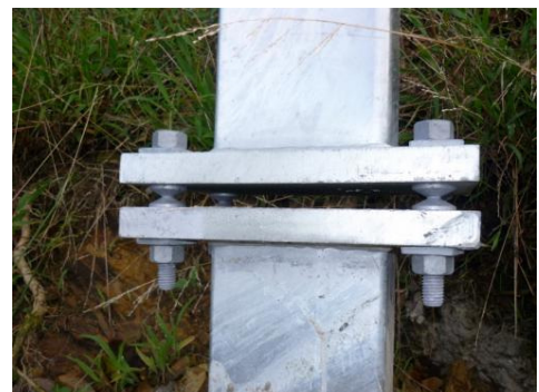
Figure 37: Breakaway/spliced pole ( left ) and slip base ( right ) [57]
