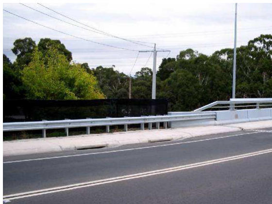
Figure 75: Transition between semi-rigid and rigid barrier [A.40]
