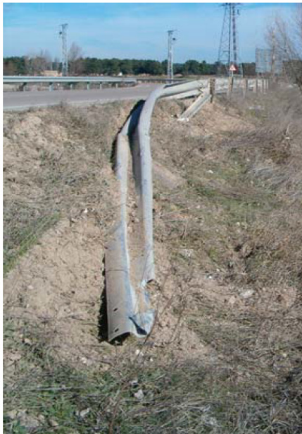
Figure 14: Result of an impact involving the first few posts of a terminal [1]
