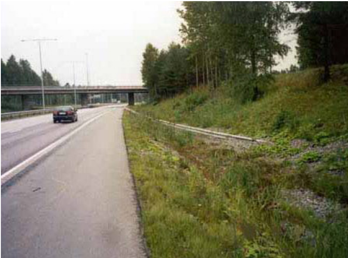
Figure 12: A buried-in-backslope terminal [1]
